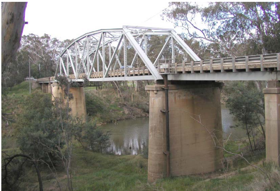
Figure 8 Bridge over the Goulburn River, Murchison
